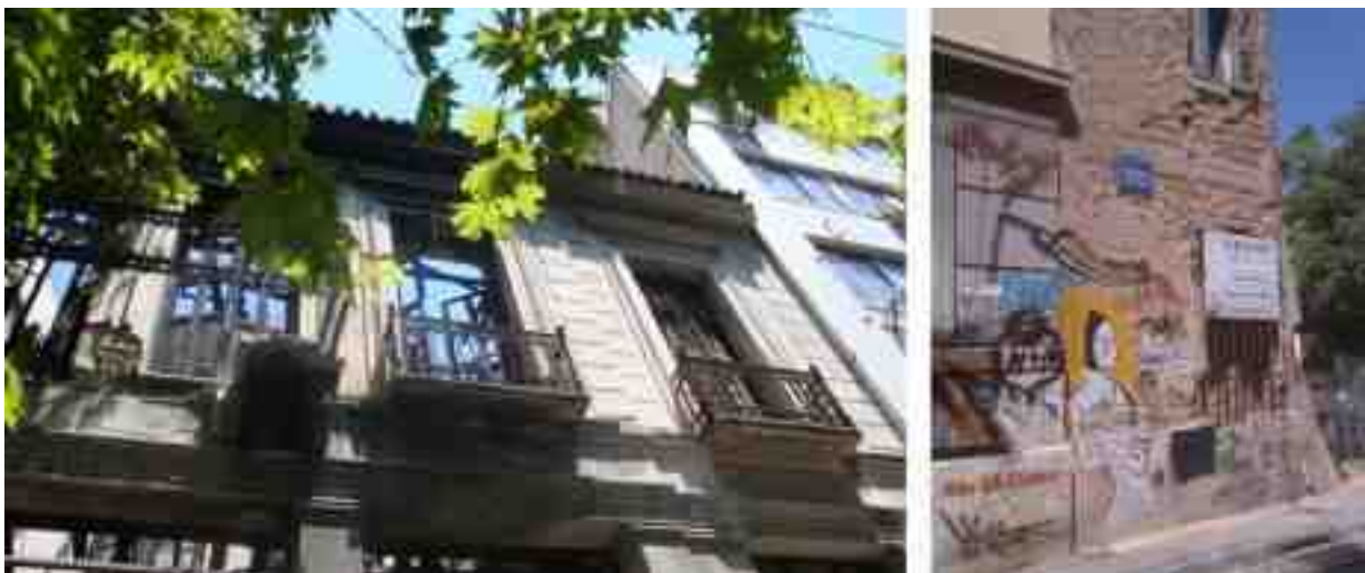
Figure 15: abandoned buildings in Gerani (Dipyliou Street).
